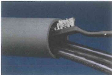
Clean duct with wire brush, solvent wipe.
