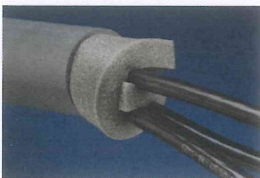
Separate cable(s) then wrap with foam strip.
