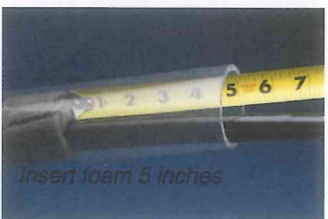
Separate cable(s) then wrap with foam strip.
